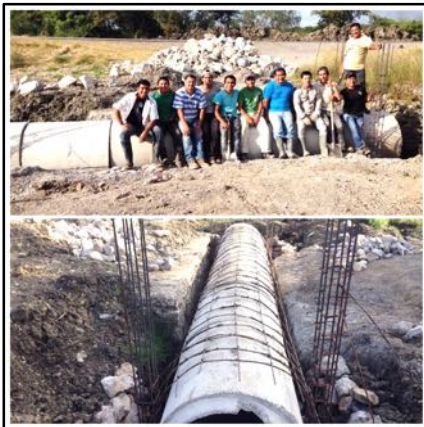
Bible College Construction New Bridge
