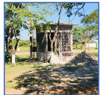
Bldg. Electrical Control
