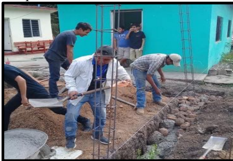
SS Classroom Construction
